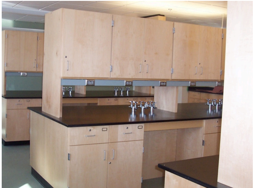
This project located in Columbia, South Carolina required an FSC Maple casework to help it achieve a SILVER level LEED certification.
